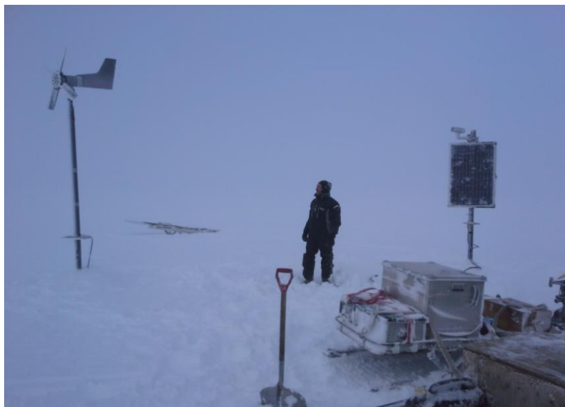
Figure 4. Photo showing the installations of the test infrastructure at the Dyngjújökull test-site in January 2014. The wind generator is mounted on a steel pipe without guy-wires, to minimize icing problems. The solar panel, web camera and communication antenna are a similar pipe 6 meters away. Between them a metal box carrying the electronic equipment is buried just under the snow.
